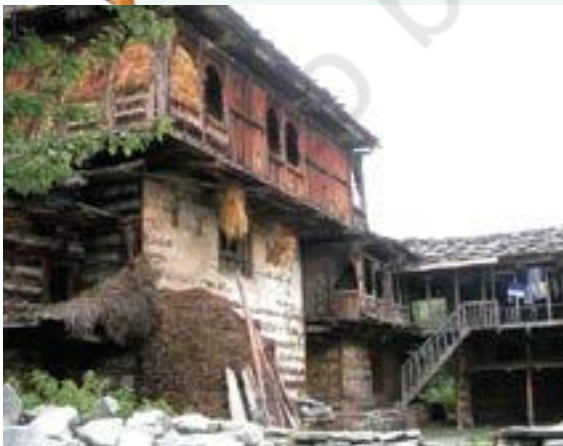
Fig. 1.6. Kath-kuni House, Himachal Pradesh
