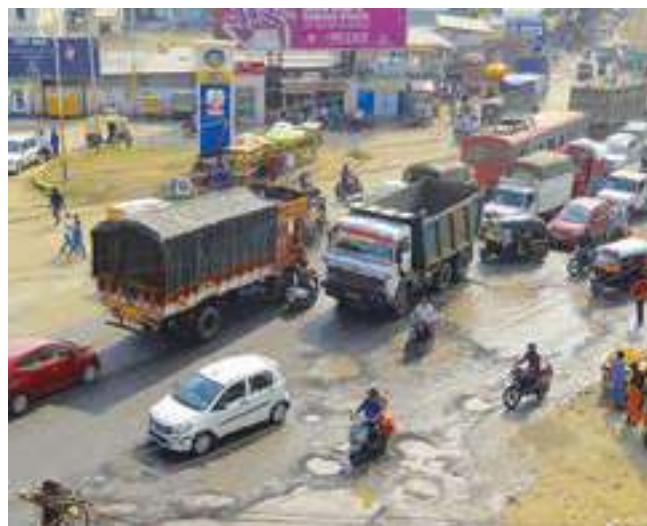
Fig. 7.27. Potholes on the roads
