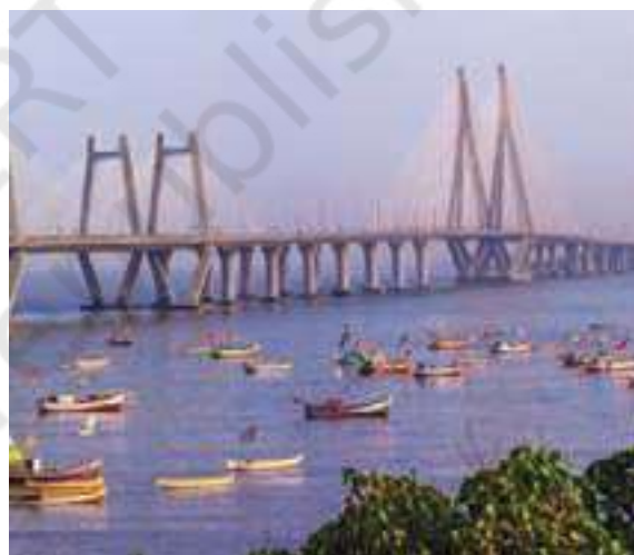
Fig. 7.10. The Bandra Worli Sea Link bridge connecting western and southern Mumbai reduces traffic jams and eases mobility for commuters
