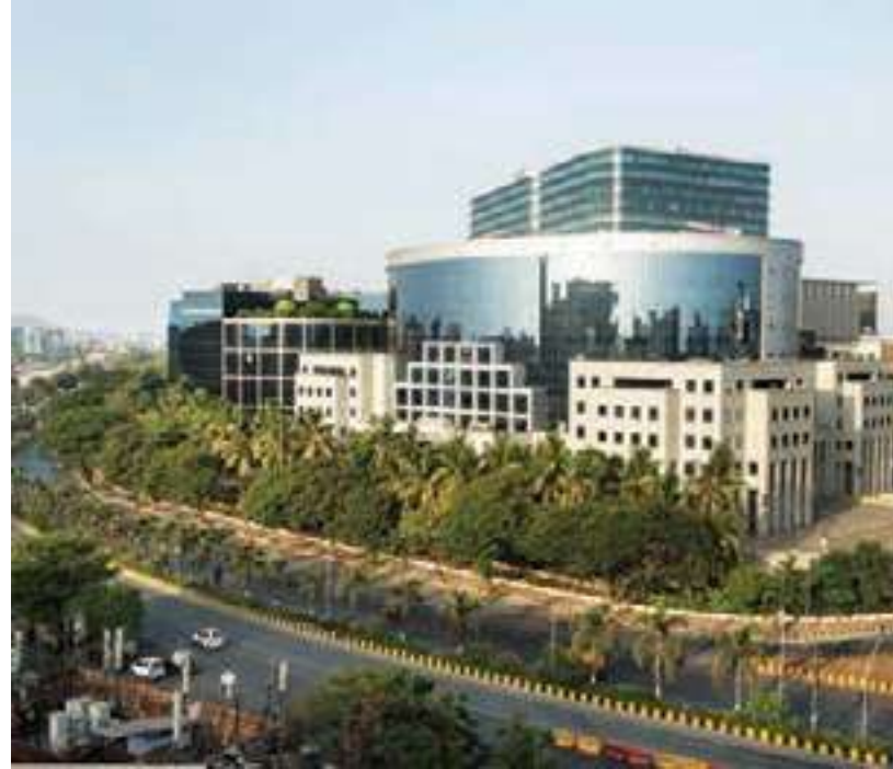
Fig. 7.12. The Bandra Kurla Complex, Mumbai, has banks, corporate offices, and financial institutions
