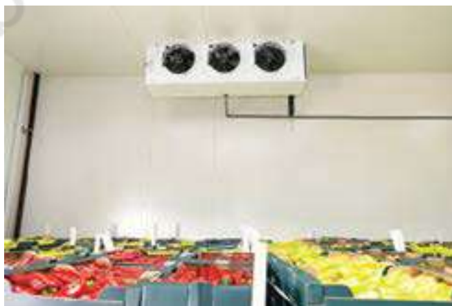
Fig. 12.12. Cold storage facility for vegetables
