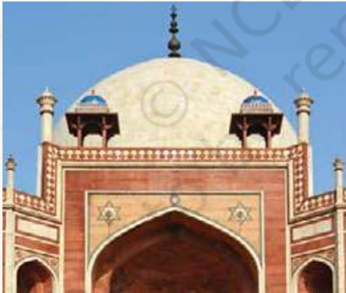
Fig. 3.42. A closer view of the upper level; note the marble domes, arches and stars.
