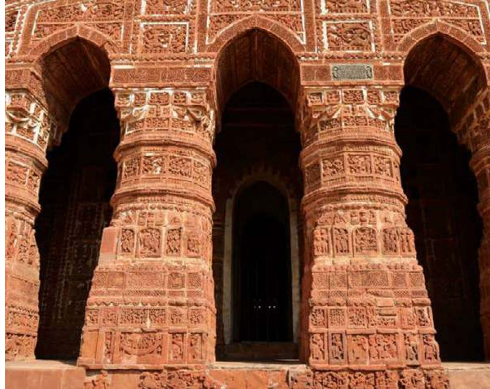
Fig. 3.27. Detail of the temple's facade (front portion), showing intricate terracotta work.
